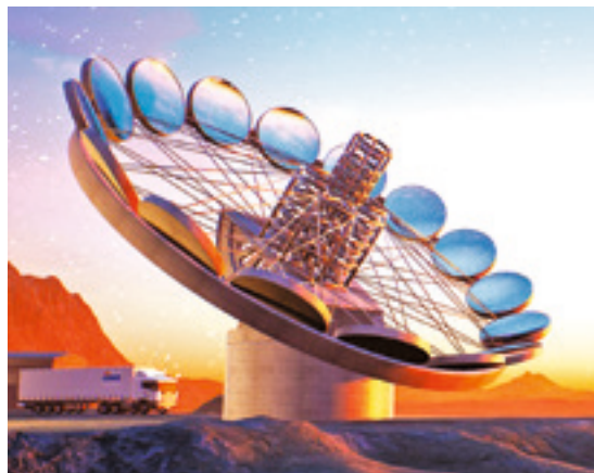
► Fig. 1: Spinning flare of e-spun polymer fibers for the fabrication of electrically conductive coatings. Fig. 2: Live-Mirror Application in a possible future telescope with an assembly of 17 mirrors with a diameter of 5 m each.
