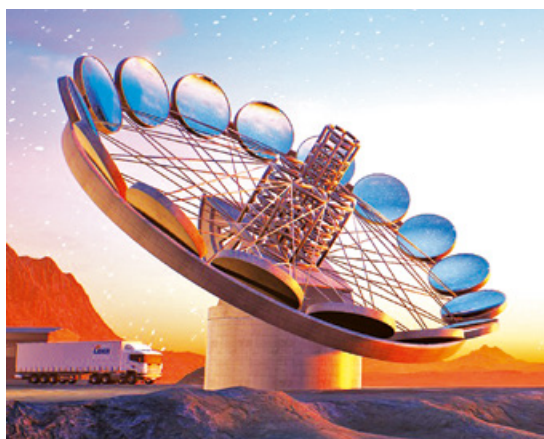
► Fig. 1: Spinning flare of e-spun polymer fibers for the fabrication of electrically conductive coatings. Fig. 2: Live-Mirror Application in a possible future telescope with an assembly of 17 mirrors with a diameter of 5 m each.
